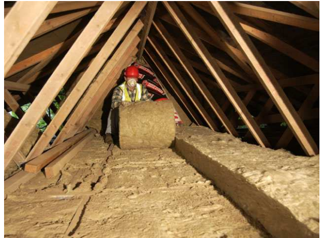
Attic insulation being installed.
